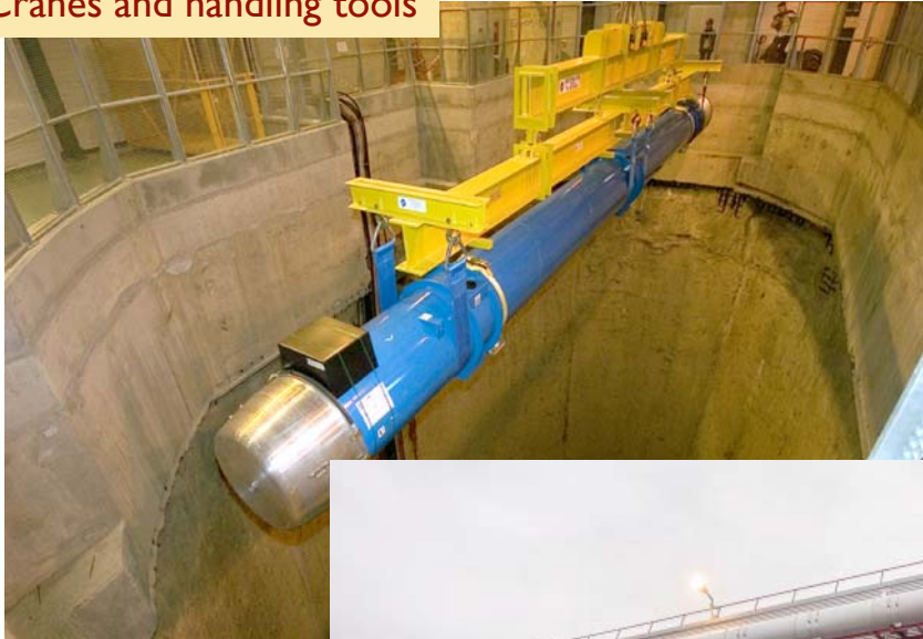
Cranes and handling tools
